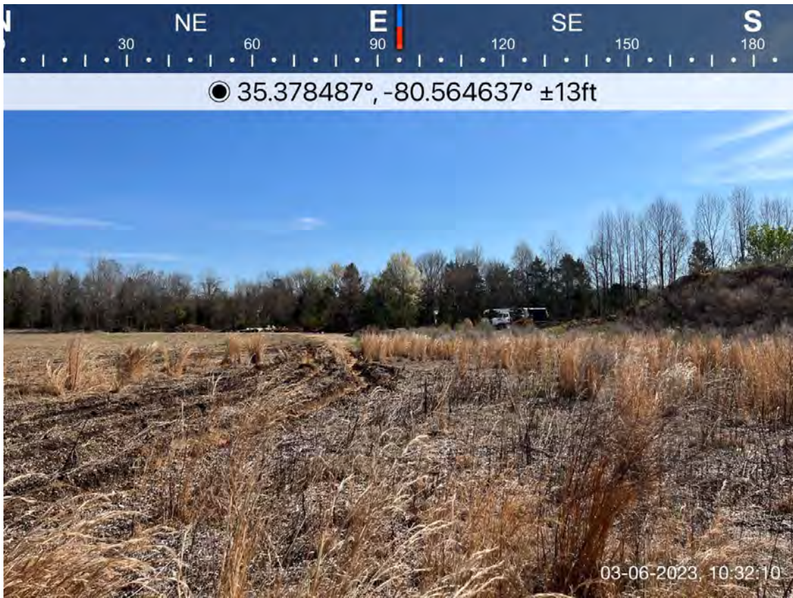
Photograph 3: Looking east across the existing grass field towards boring S-5 and spoils piles.
